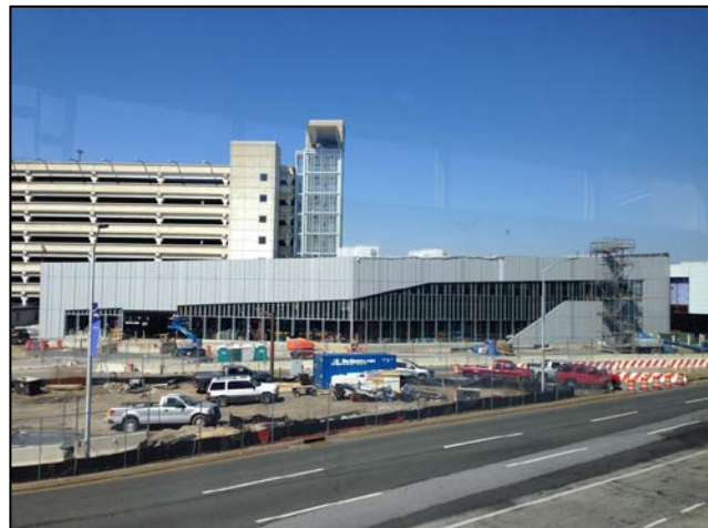
Terminal F Baggage Claim Building Under Construction
