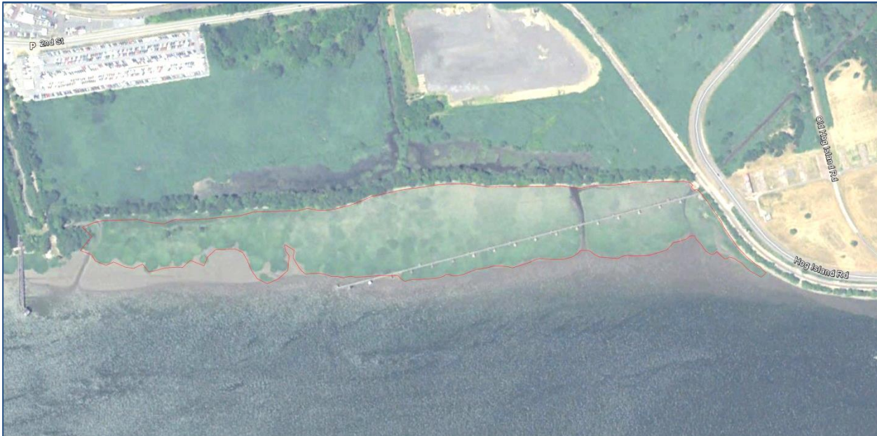
Aerial 1: Project area captured at low tide, exposing the extent of regulated tidal wetlands, shown outlined in red. Total area is approximately 20 acres. (Source: Google Earth 9/1/2010). Mean low water is at elevation -2.36.
