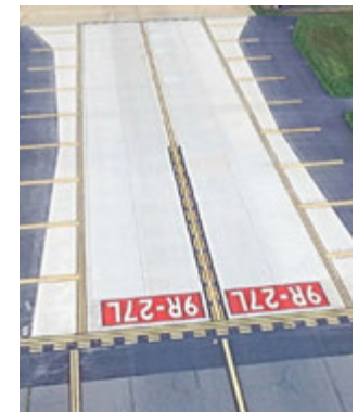
Figure 22. Taxiway U & Y Rehabilitation Project
